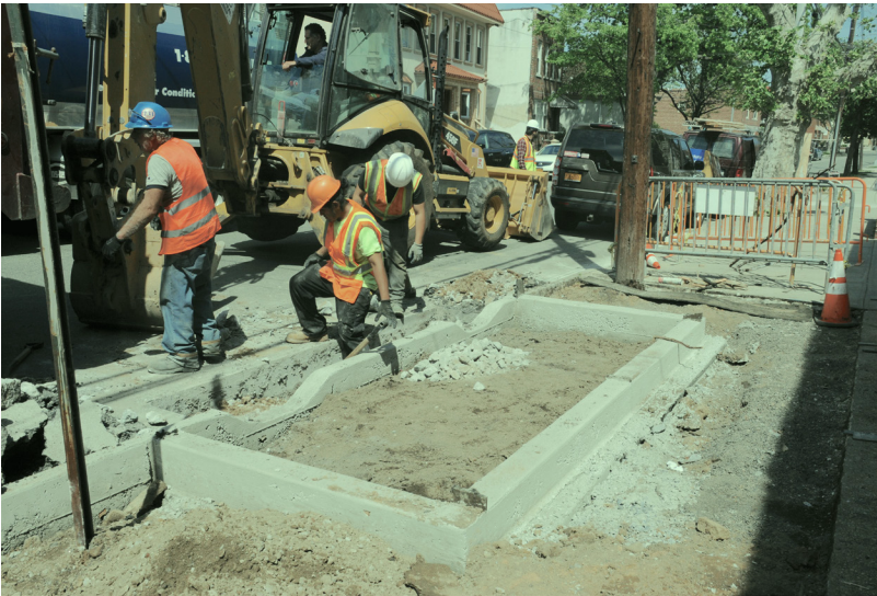
Construction of bioswales in Queens. Source: NYC-DEP
