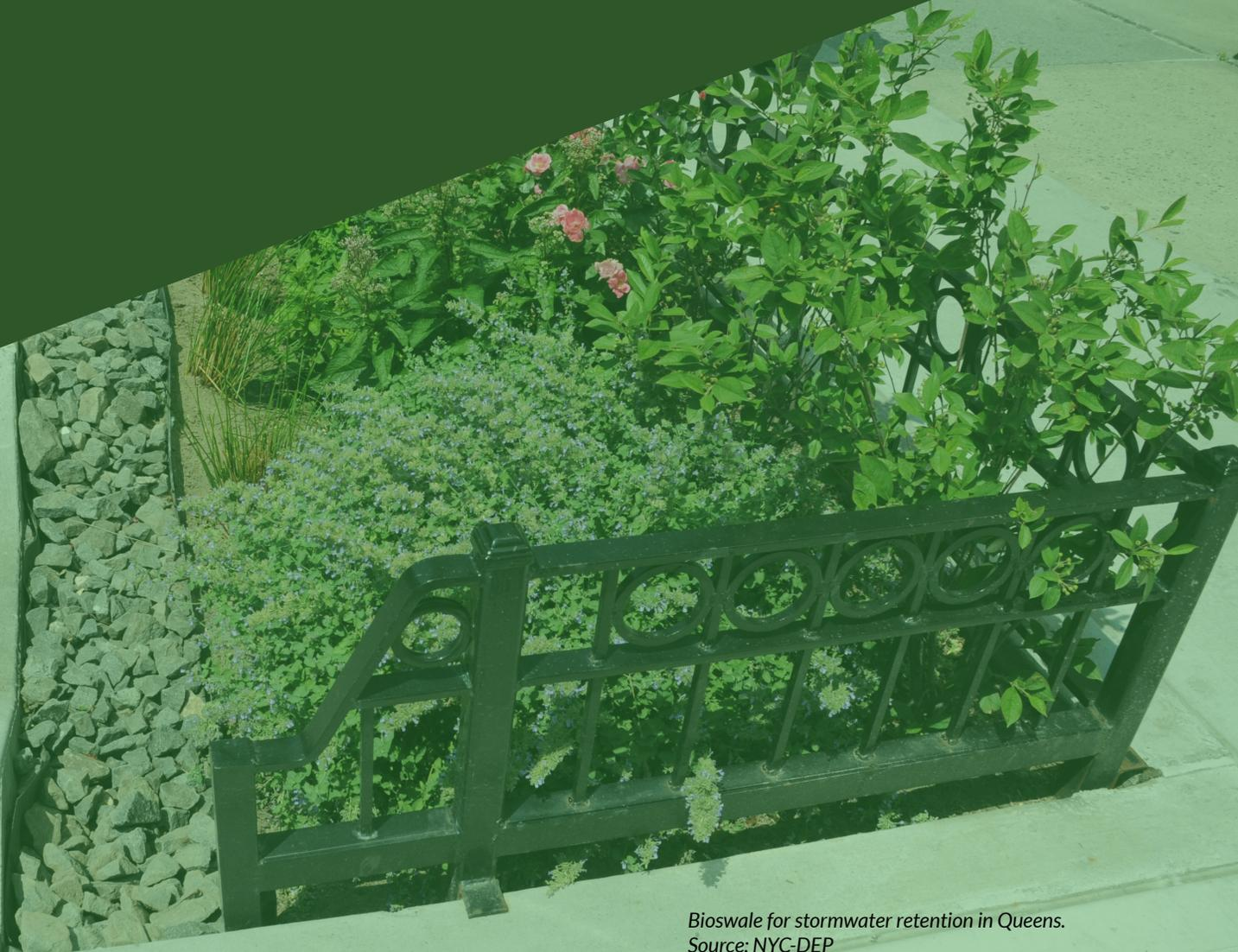
*Bioswale for stormwater retention in Queens.
